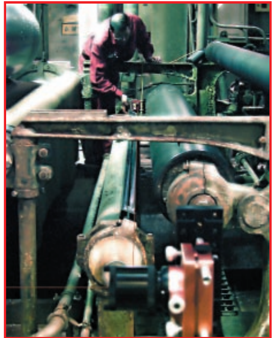
Roll parallel measurements being done by plant maintenance personnel during an unscheduled outage.
